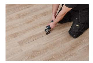
Adjust circular saw to the depth of the LVT board and cut the plank lengthwise along its center axis;
