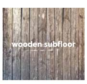
Check the floor for insect infestations. Make sure the subfloor is levelled and screw down any loose sections firmly. Wooden subfloors should always have access to air and should be ventilated at the edges. If there is any moisture in the woodbased subfloor or there is no proper moisture barrier below the wood-based subfloor, it must be removed first.
