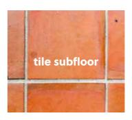
Check the subfloor for moisture problems. The joints of the new floor covering should never be aligned with the underlying tile joints. It is not necessary to fill the grouts of a subfloor comprised of ceramic tiles with joints when these do not exceed 5 mm in width. Bear in mind that some ceramic tiles may show rising edges/corners although the main level may be correct. These parts may telegraph through the floor covering in the future.
